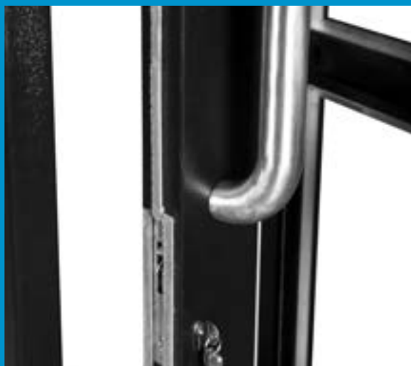
STAINLESS STEEL PULL HANDLE AND MORTICE LOCK
